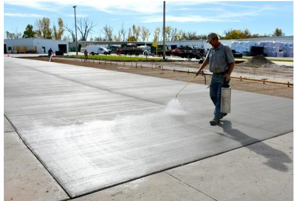
PENCURE OTC offers multiple features including a simple, single-step application method. It minimizes crazing and shrinking cracks common to improperly cured or uncured concrete. PENCURE OTC complies with ASTM C309, Type 1, Class A and B. Its permeable film allows moisture in cured concrete to evaporate. PENCURE OTC provides a low-gloss, satin appearance. It is a clean membrane that will not yellow.
